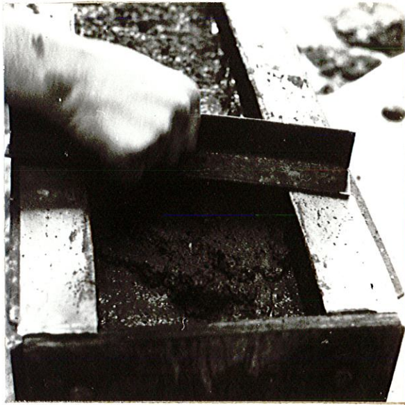
Figure 3. Screed used to level concrete
